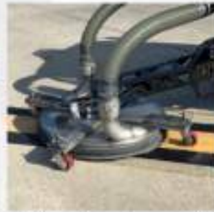
Paint Cleaning and Rejuvenation
